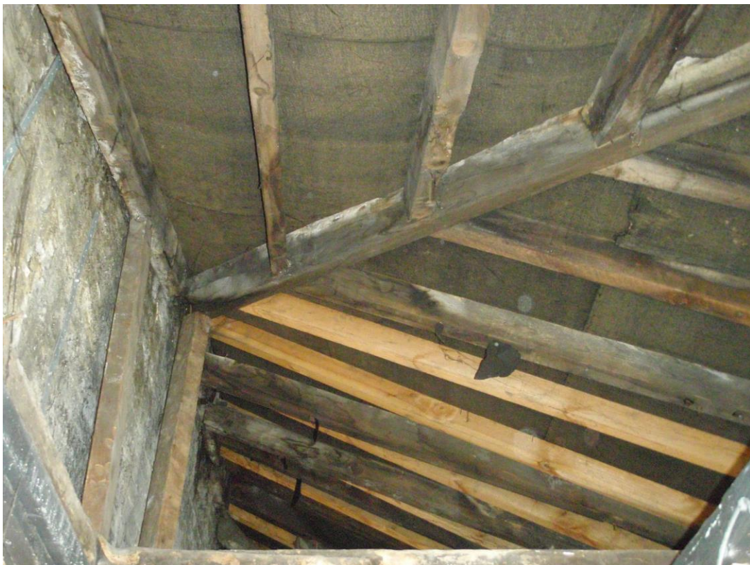
Plate 12. Soot blackened roof timbers of Unit 21B
