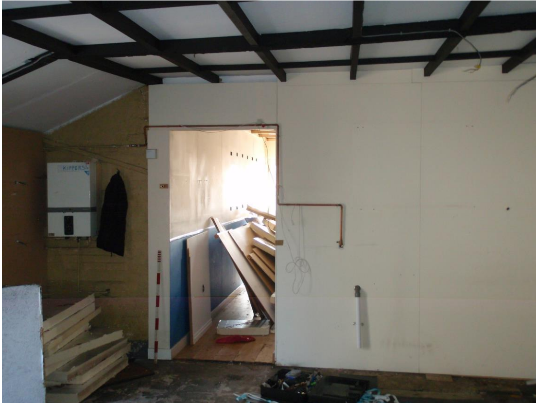
Plate 8. Interior view of Unit 21B (looking south)
