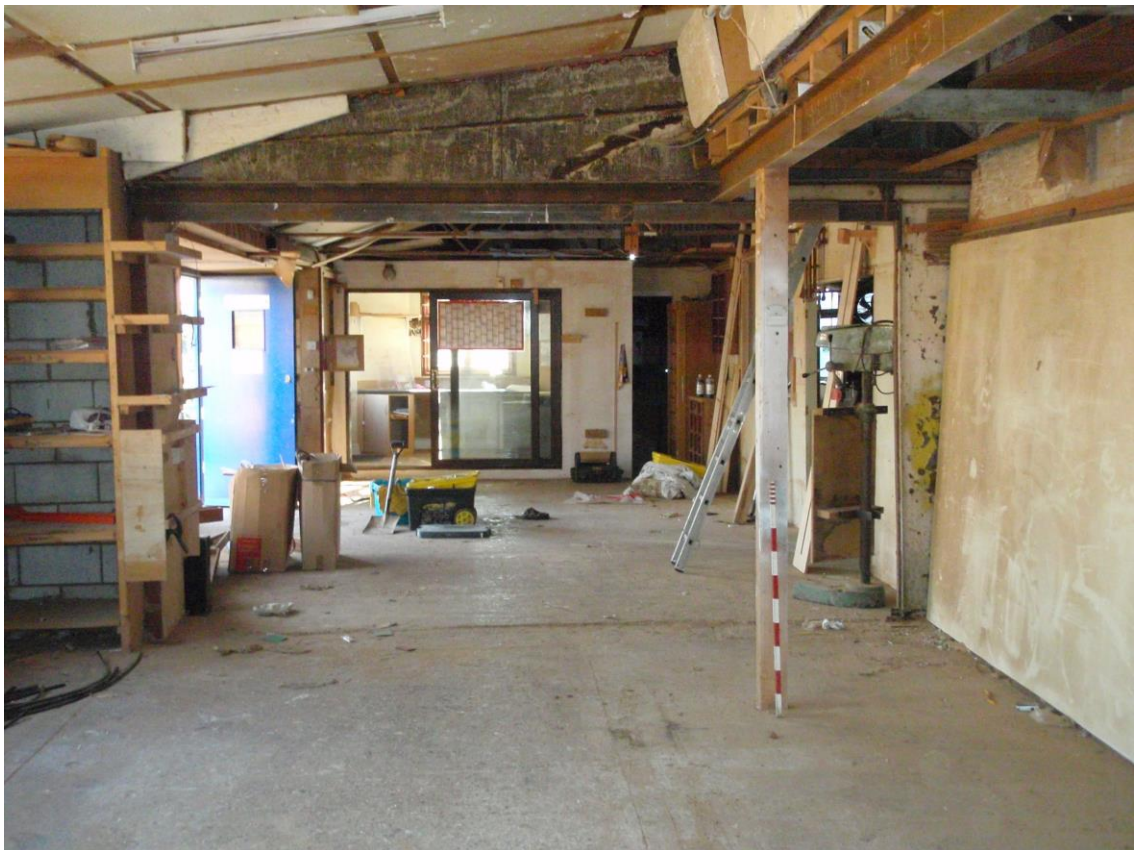
Plate 2. Interior of Unit 21A (looking south)
