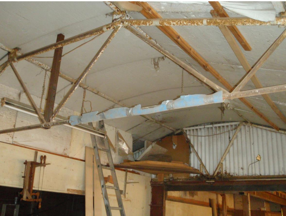
Plate 4. View of roof trusses Unit 21A
