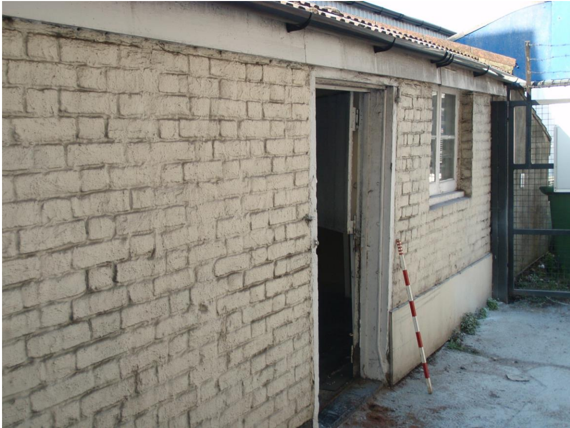
Plate 5. Exterior east facing wall of Unit 21B
