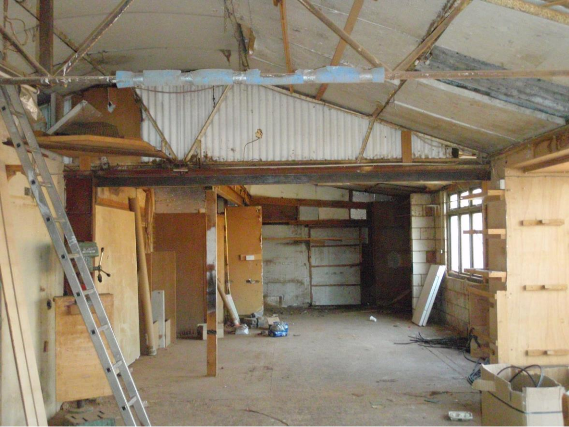
Plate 3. Interior of Unit 21A (looking south)
