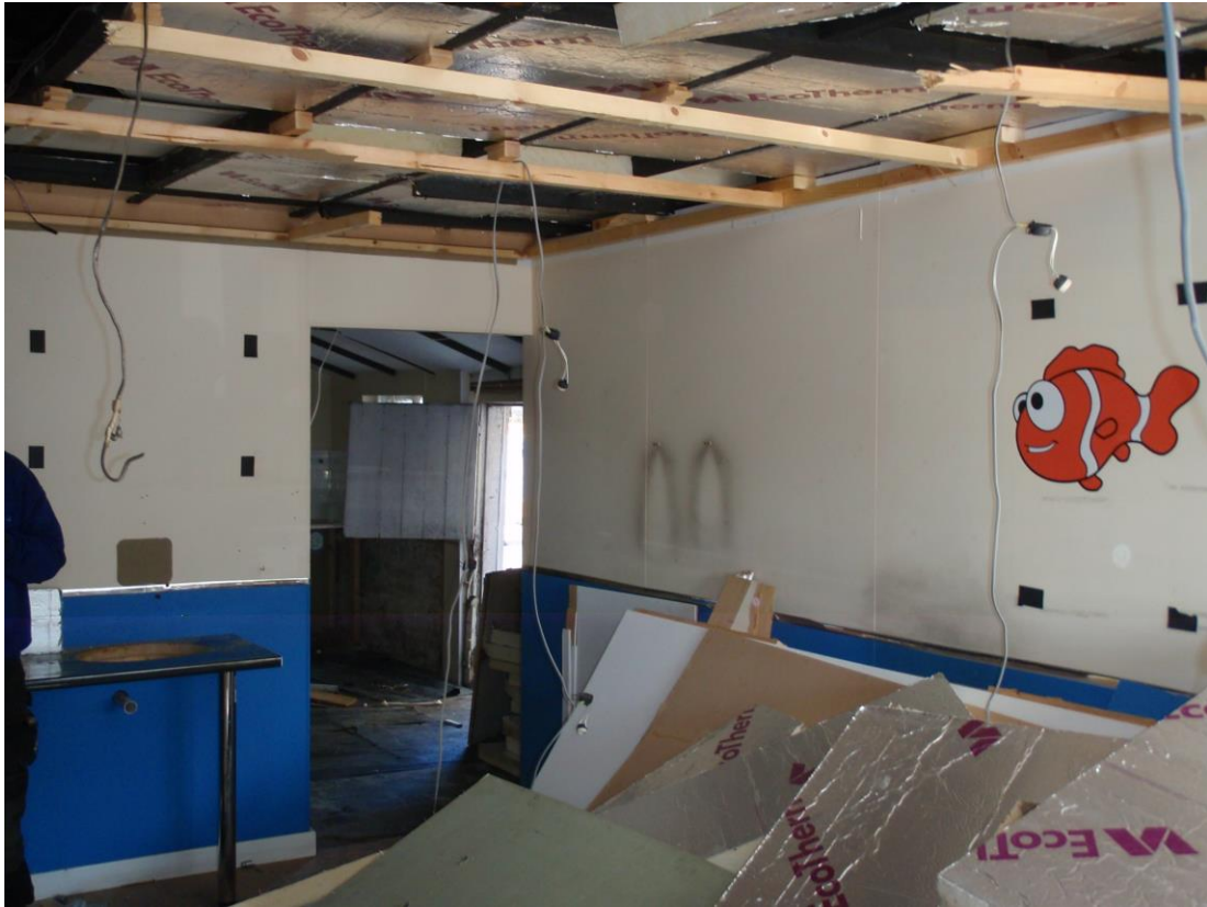
Plate 11. View of interior of Seafood Shop (Unit 21B)
